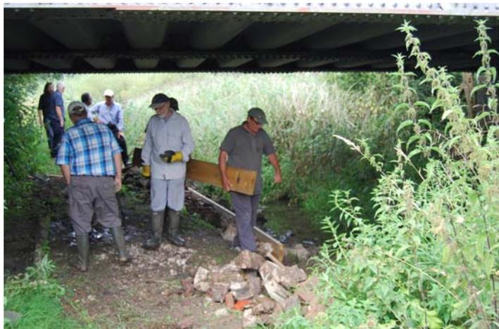
Shuttering cut to size and ready to put in place, you can see the size of the rocks that were removed in the foreground
